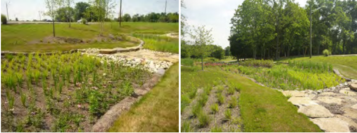
Figure 124. Bioretention Basins (stormwater.wef.org)
