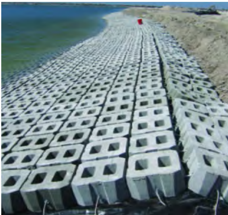
Figure 5. Articulated Concrete Blocks Example (Acfenvironmental.com)
